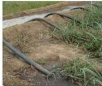
Siphons at work at Manyonyo
