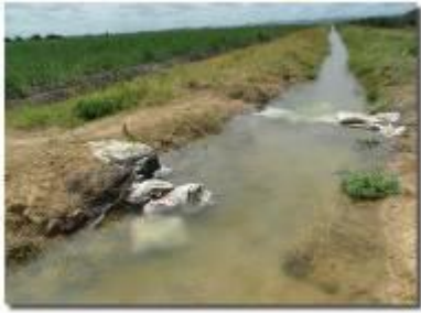
Not ideal: Makeshift control structures in Manyonyo
