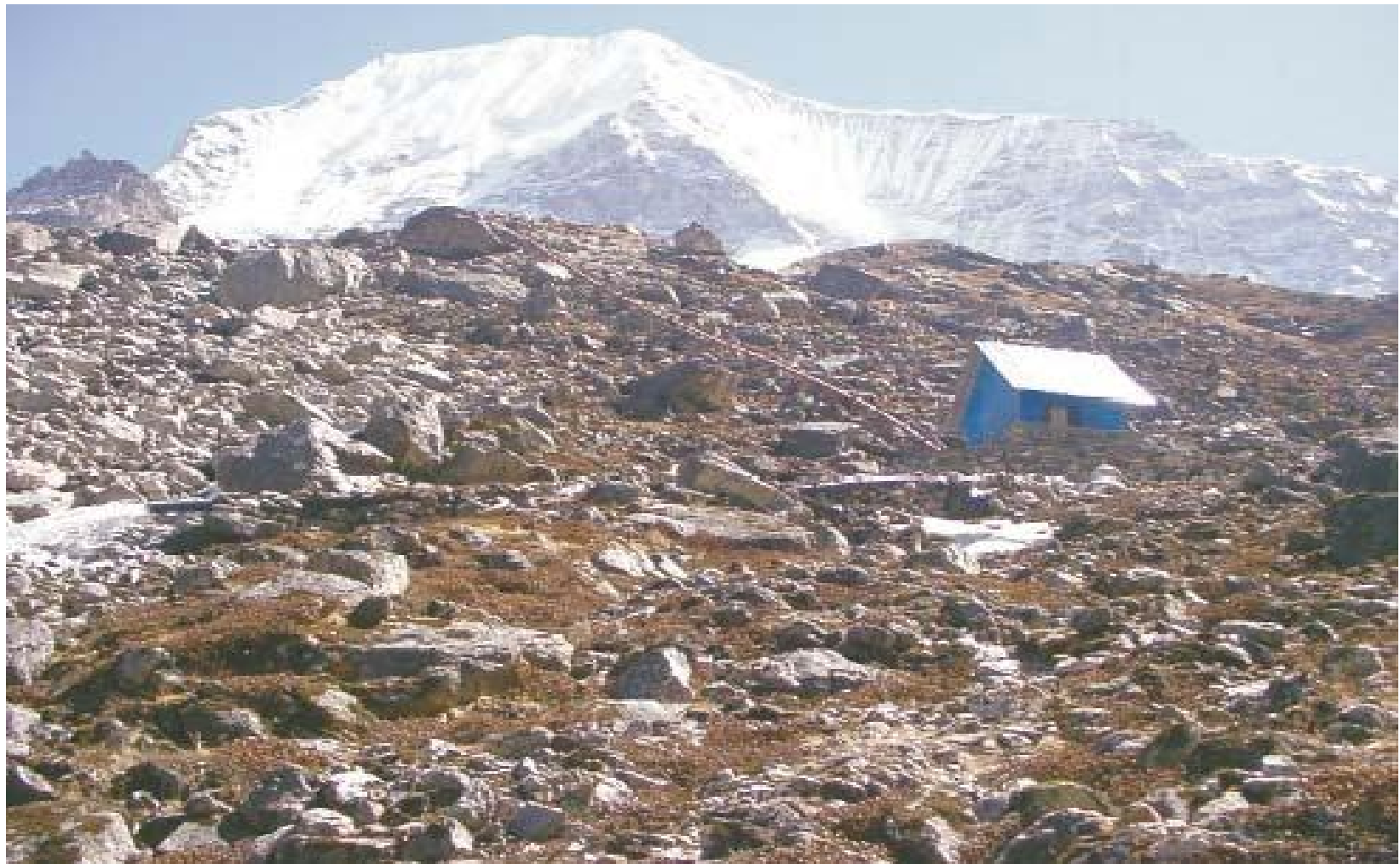
Highest micro hydro powered plant TShO Rolpa Approx 4500 meters
