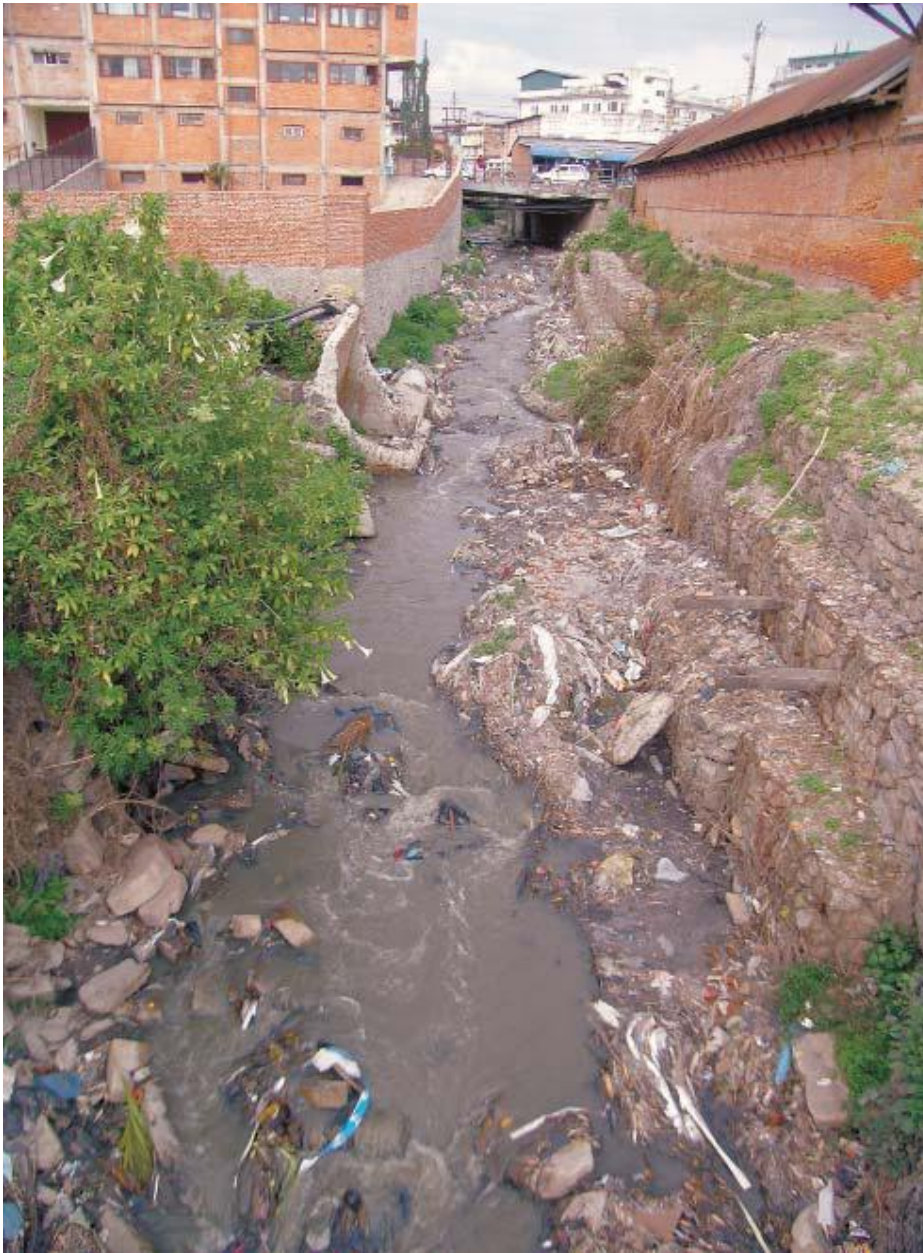
Stream changed in to sewer in Kathmandu
